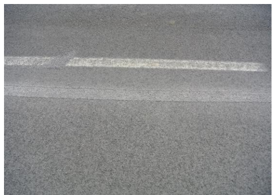
Treated construction joint
