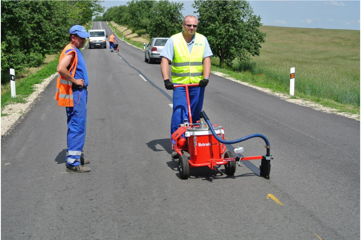
Treating the construction joint with Rissflex and a rubber spreader
