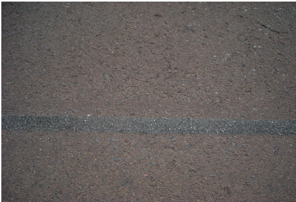
The crack after it has been treated with Rissflex
