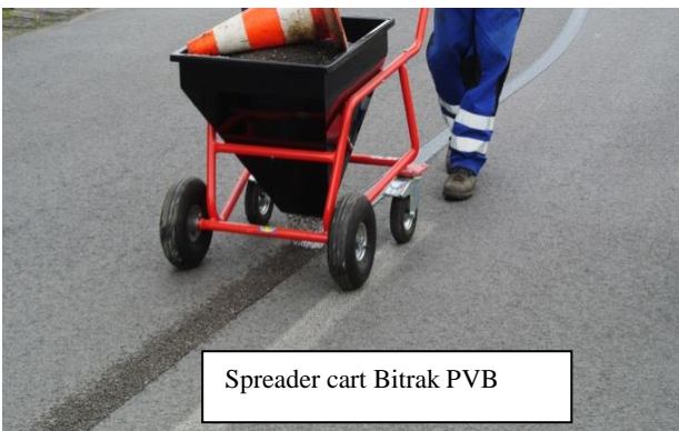
Spreading the treated joint with crushed aggregate
